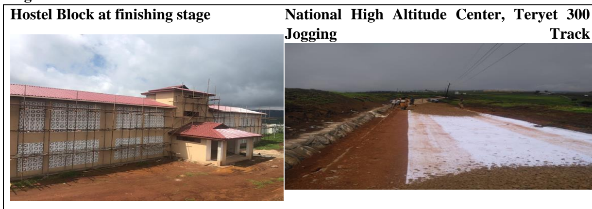
Figure 2.3: Civil works at the Hostel
